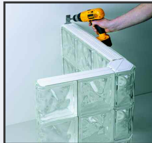
3 » The glass blocks are secured to the wall using special wall anchors.
