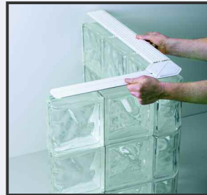
2 » Place the horizontal, vertical and specialty shaped spacers on the silicone to align and keep each row of blocks perfectly in place.
